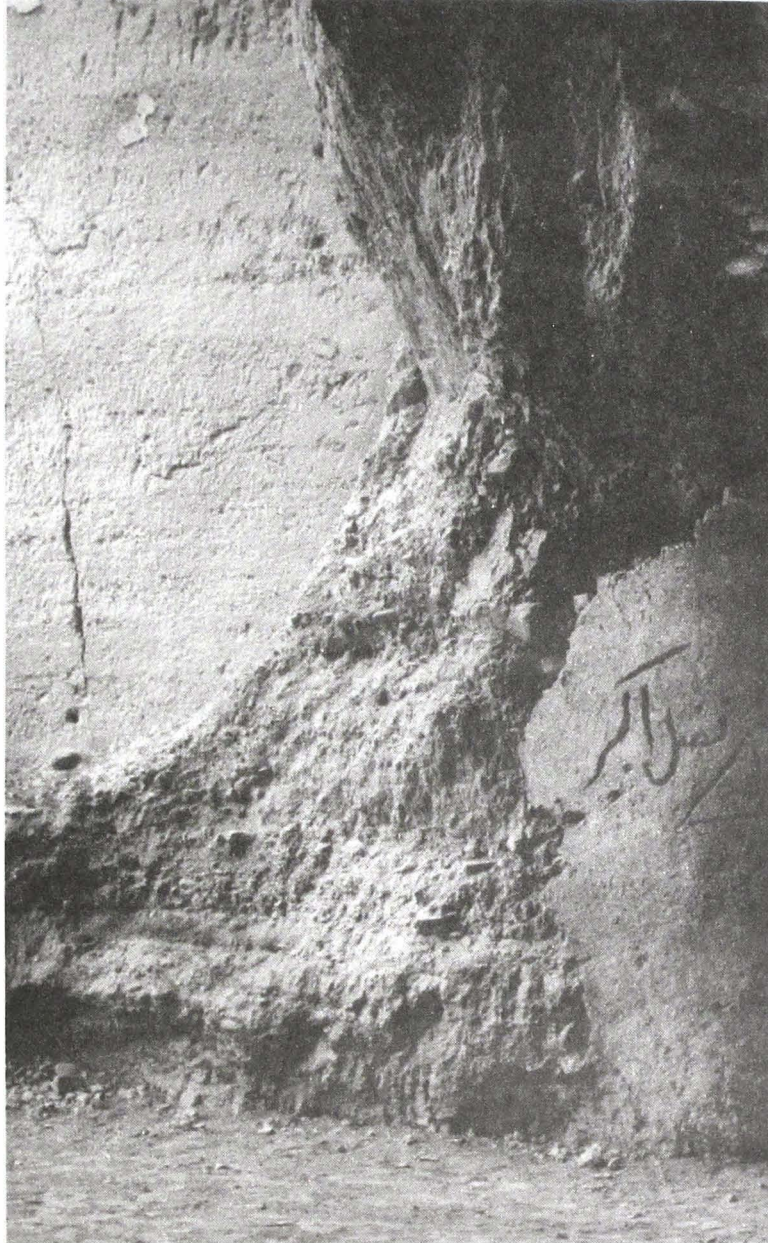
16. The damaged heel of the right foot of the Big Buddha.
